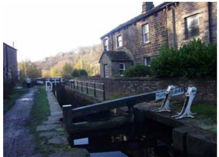
Inclined paddle gear on the Diggle Flight and beams on the non-towpath side
